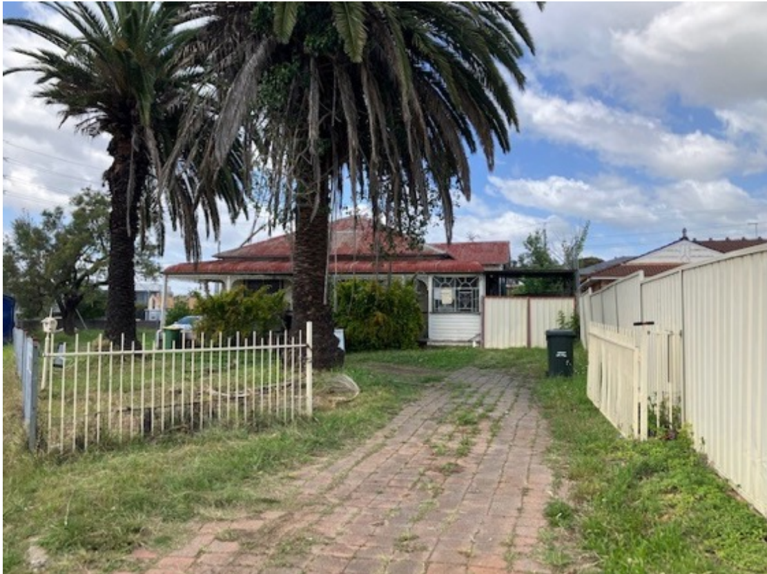
Figure 26: Looking south from Cabramatta Road East towards the dwelling.
