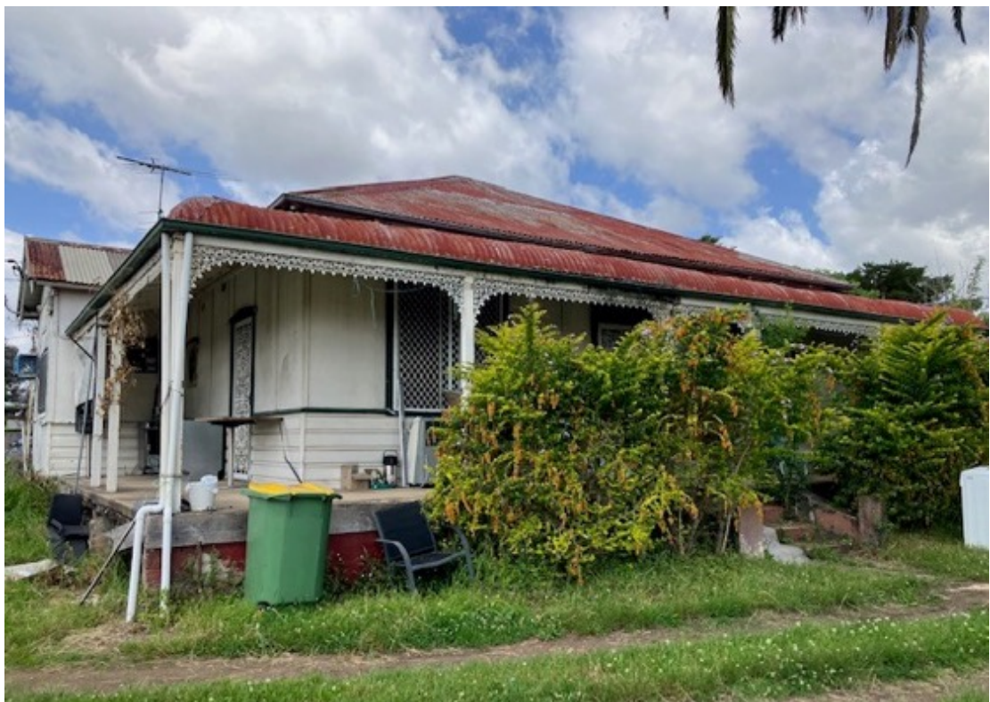
Figure 27: Looking at the north-eastern corner of the dwelling. The south-eastern wing with striped corrugated roof, gable end and Inter-War style chimney (not visible) evident in the background.
